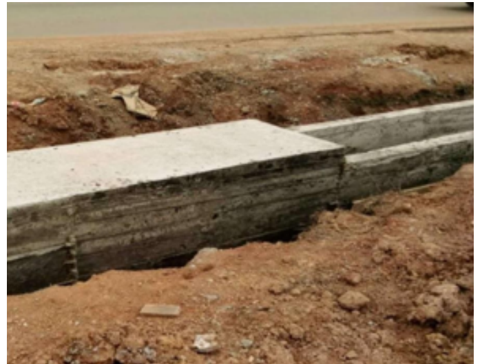
CONSTRUCTION OF 0.6 X 0.6 U DRAIN AT WENCHI
