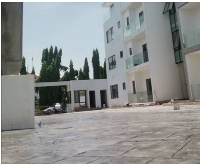
STAMPED CONCRETE WORKS
