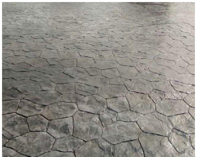
STAMPED CONCRETE WORKS
