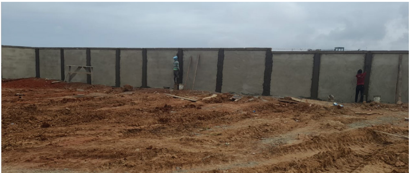
DESIGN AND CONSTRUCTION OF FENCE WALL AT CANTONMENTS LENGHT OF WALL - 129m
