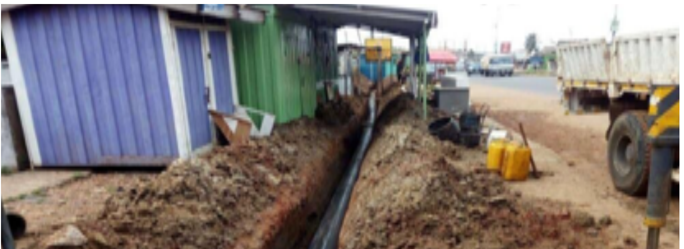
LAYING OF HDPE PIPE AT KUMASI
