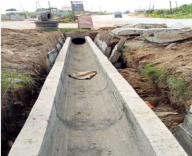
CONSTRUCTION OF 0.6 X 0.6 U DRAIN AT WENCHI
